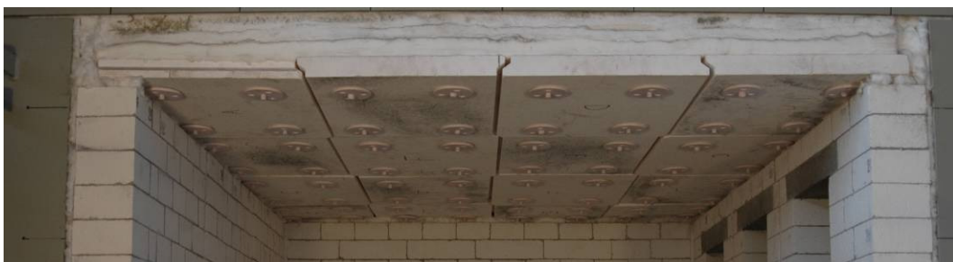
The Lite-Cell roof after the installation
