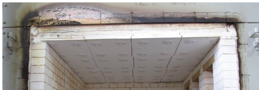
The Lite-Cell roof after 18 months of operation
